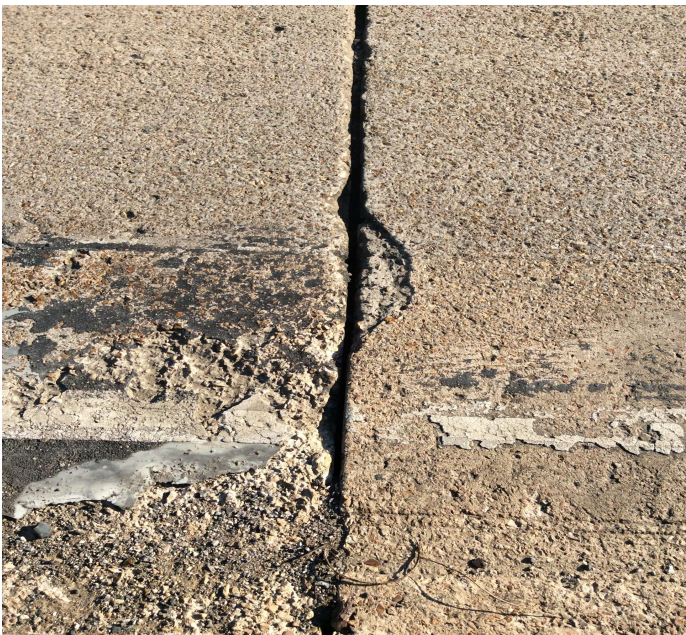
PHOTO 1 Description Joints are cracked, deteriorated & filled with debris at Bents 2, 4, 6, 8, 10, 12, 14, and 16.
