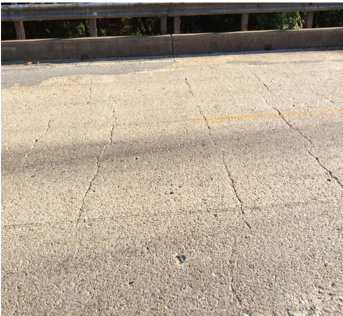
PHOTO 1 Description Span 1. Typical of unsealed cracks to deck at all spans.
