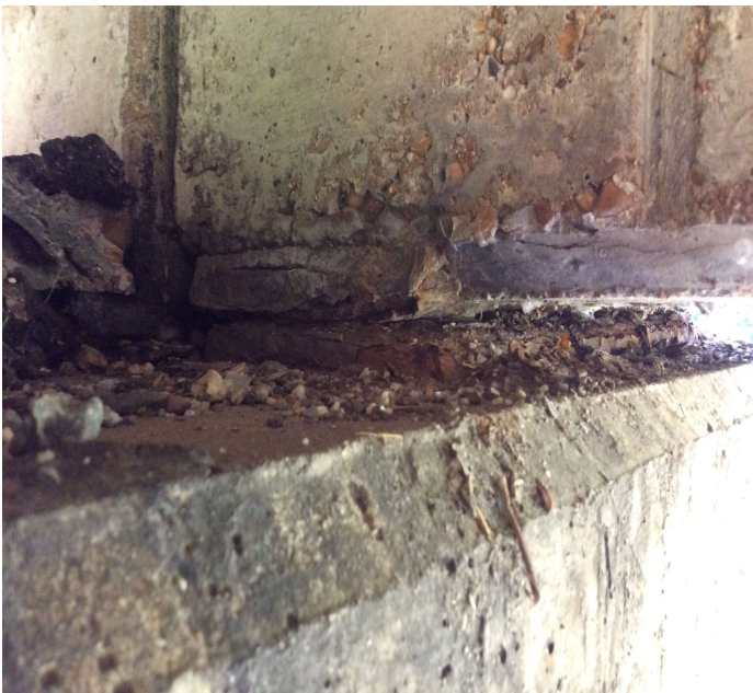
PHOTO 1 Description Bearing assembly below Girder 6. Typical of rust to Bearings 1 & 6 at Bents 2, 4, 6, 8, 10, 12, 14, and 16.
