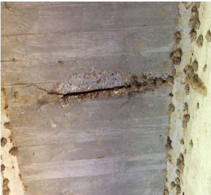
PHOTO 1 Description Span 3 between G4-G5. Typical of spalls to deck below, some with rebar exposed at all spans.
