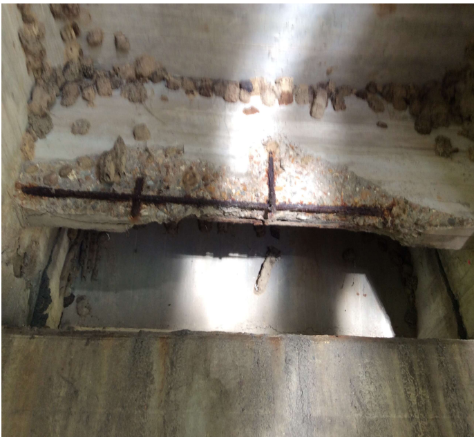
PHOTO 1 Description Typical diaphragm at G3 - G4 at Bent 2. Spalls with rebar &/or cracking to concrete diaphragms at Spans 5 - 8 & 10 - 14 & 17.
