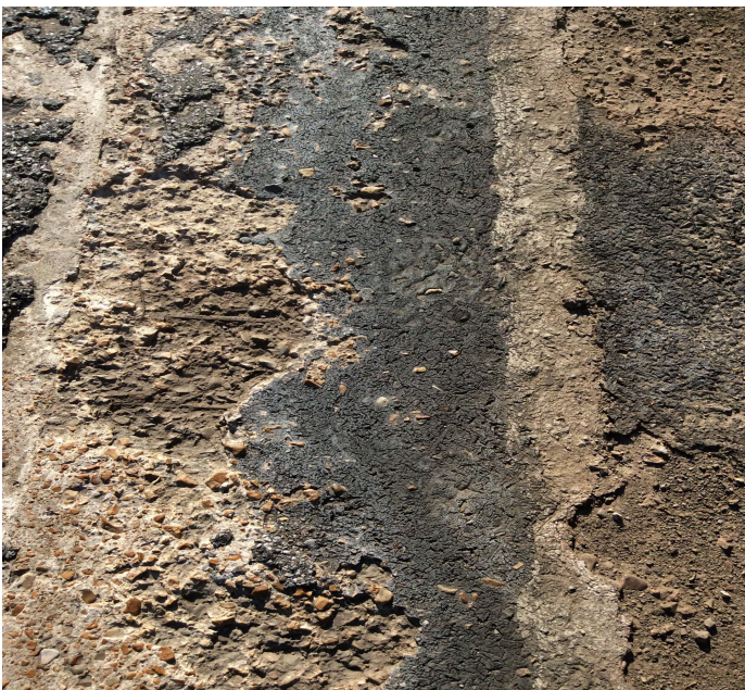
PHOTO 1 Description Area of deterioration & scaling w/t rebar exposed in right gutter line at Span 8.
