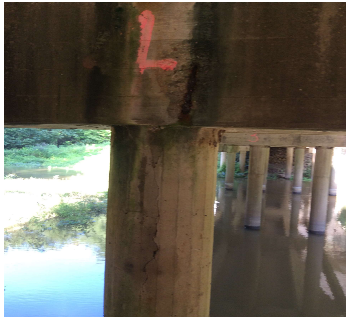
PHOTO 1 Description Pile 4 at Bent 4. Typical of spalls with rebar exposed &/or cracking to concrete piles at Bents 2, 3, 4, 8, 10, & 11.
