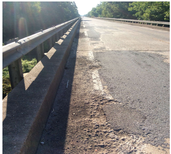
PHOTO 2 Description Deterioration & Scaling of gutter on left side, typical of Left & Right.
