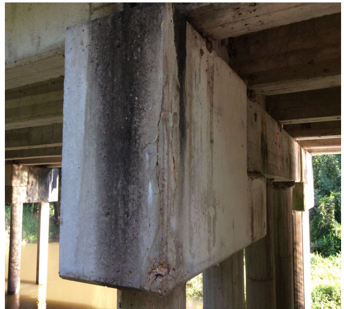
PHOTO 2 Description Crack on Right end of cap at Bent 3. Cracks & Spalls with rebar exposed to caps at Spans 2 - 6 & 8 - 16.
