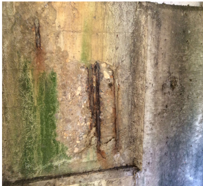
PHOTO 1 Description Cracks & Spalls with rebar exposed to cap at Spans 2 - 6 & 8 - 16.
