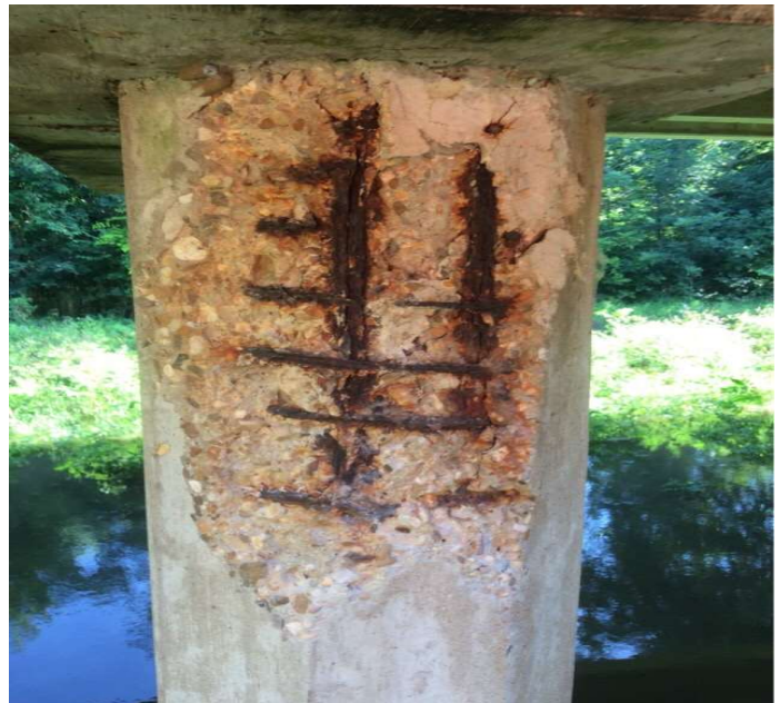
PHOTO 2 Description Pile 6 at Bent 8 with section loss to rebar. Spalls with rebar exposed &/or cracking to concrete piles at Bents 2, 3, 4, 8, 10, & 11.
