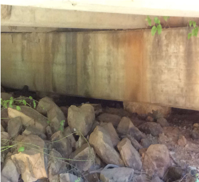
PHOTO 1 Description Photo at Abutment 2. Embankment has settled at Abutment 1 & 2 with 2 piles exposed at each abutment.
