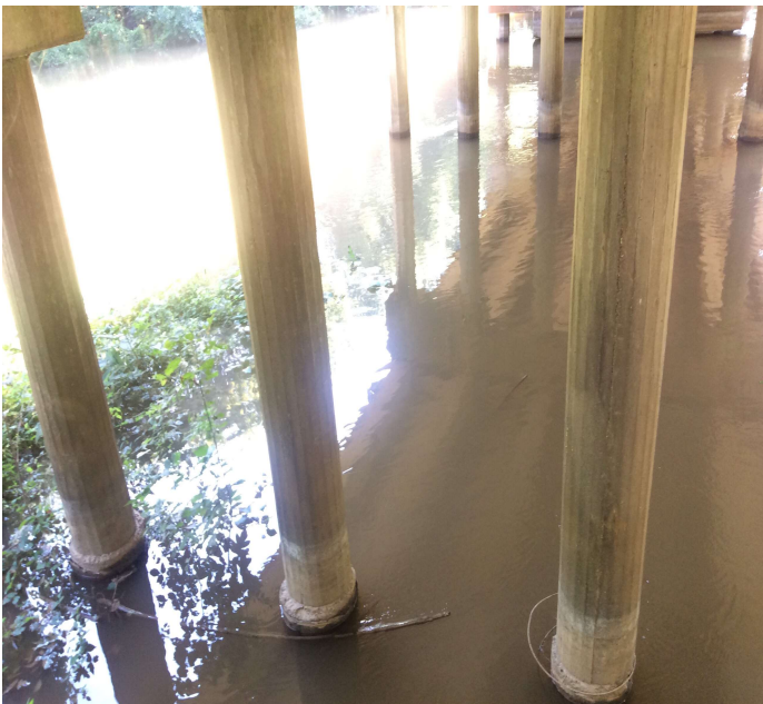
PHOTO 1 Description Typical of scour at Bents 1, 2, 4, 9, 10, 11, 12, 13, 14, 15 & 16.
