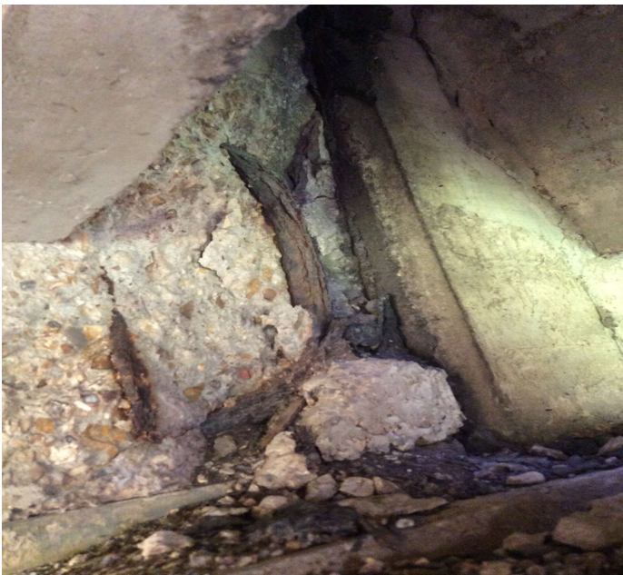
PHOTO 1 Description Girder 5 at Span 2. Typical of spalls with rebar exposed to girders at Spans 2 - 17.
